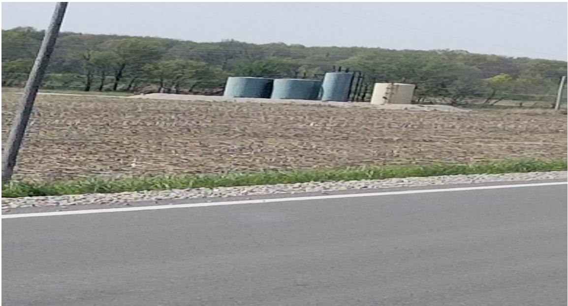
Figure 19.0. Typical Storage tanks for Pump Jack
