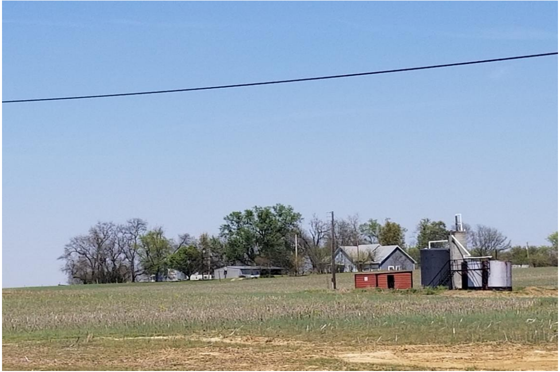
Figure 16.0. Water and Oil storage tanks located in Pump Jack field.
