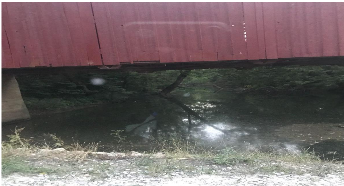
Figure 12.0. Underneath the Red Covered Bridge
